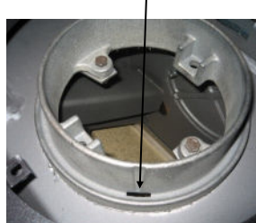
A condensate drain has now been made.
