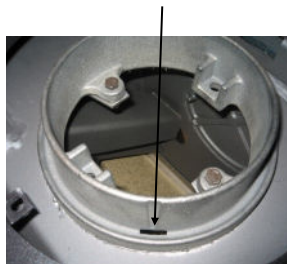
A condensate drain has now been made.
